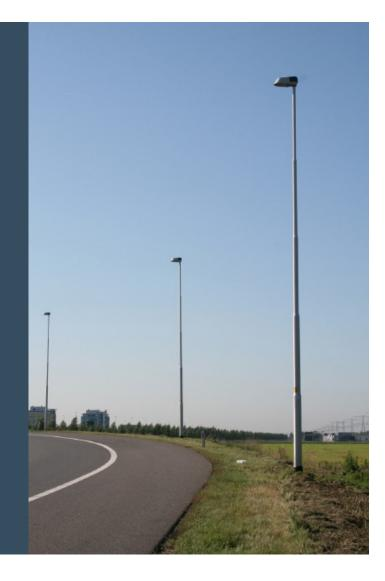
Low energy (LE) absorbing poles are generally designed to bend in front of and under the impacting vehicle before shearing or detaching toward the end of the impact.
